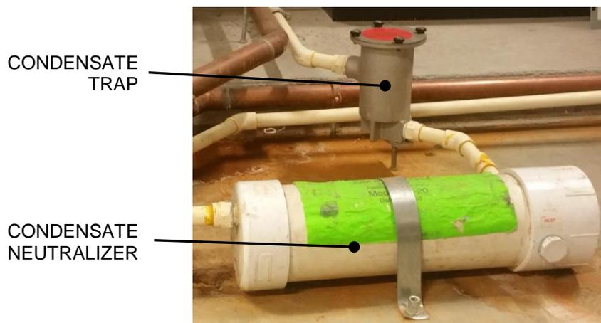
**Figure 8-7: Condensate Trap and Neutralizer**
