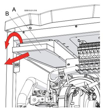
Figure 17-9 Remove the air filter "B"
