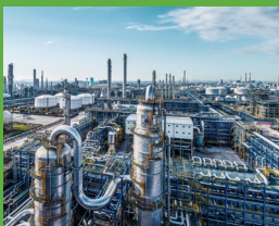
District energy plants
