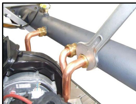
Figure 7: Removing the Gas Pipes from Gas Manifold
