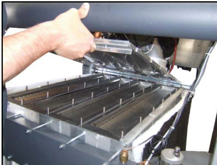
Figure 11: Lifting Burner Plates (Left) to Expose Burner Modules (Right)
