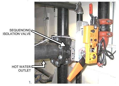
Figure 2-19: Sequencing Isolation Valve Installed
