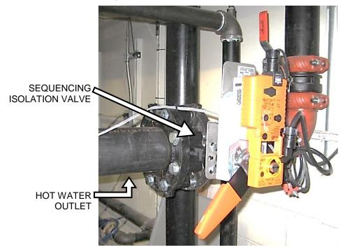
Figure 2-19: Sequencing Isolation Valve Installed
