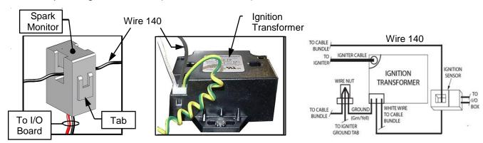
Figure 7-11: Spark Detector Sensor (AC Current Transducer) P/N 61034
