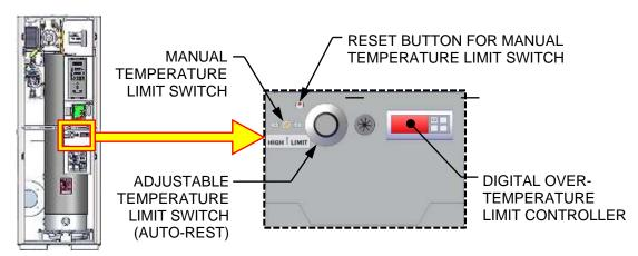
Figure 4-6a: BMK 750 & 1000 Over-Temperature Limit Switch Location
