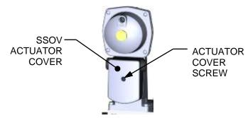
Figure 5-9: SSOV Actuator Cover Location
