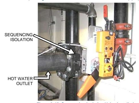
Figure 2-15: Sequencing Isolation Valve Installed
