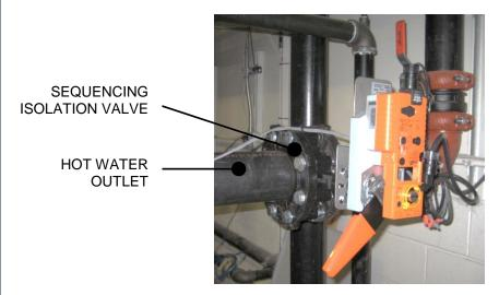
Figure 2-13: Sequencing Isolation Valve Installed
