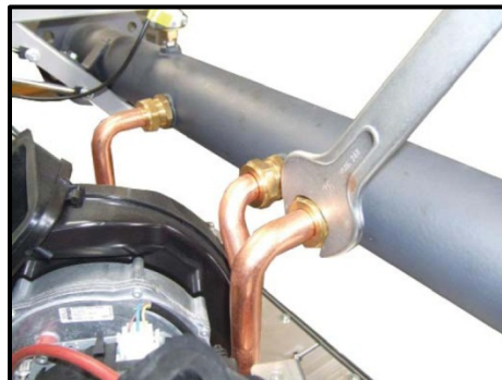
Figure 8-12: Removing the Gas Pipes from Gas Manifold (Step 8)
