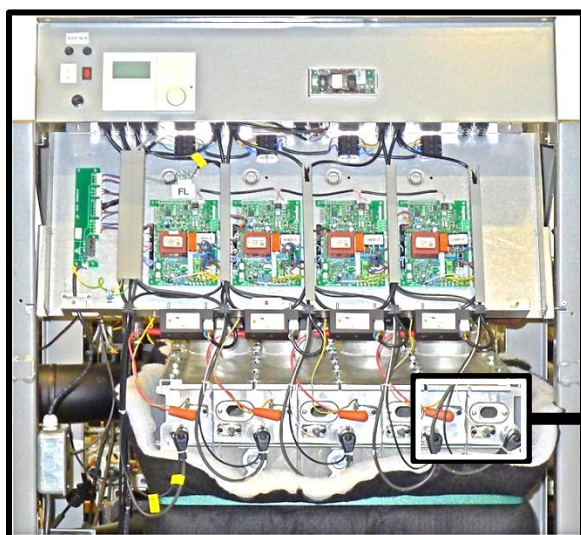
Figure 8-2: Boiler Flame Observation Port Location
