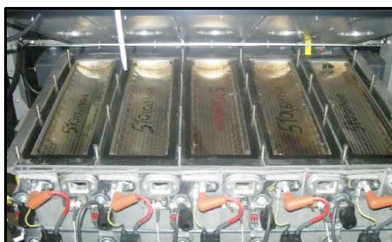
Figure 8-23: Burner Modules Exposed for Cleaning
