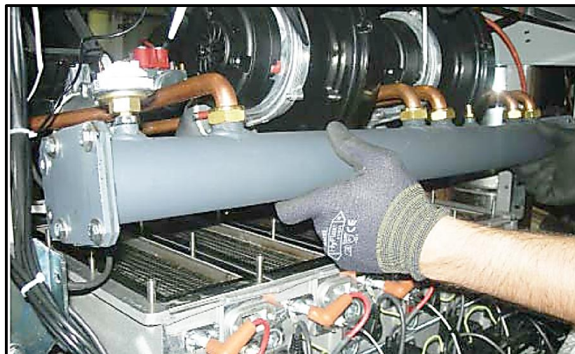
Figure 8-20: Lifting Burner Assembly from Front (Step 15)
