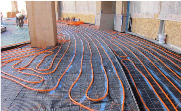
Watts Radiant® and SunTouch snow melting systems
