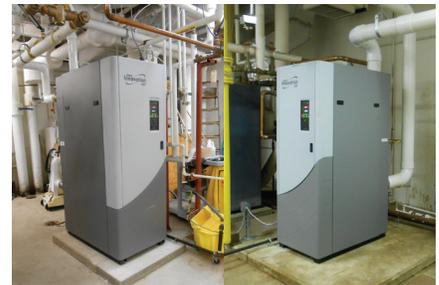
The 1,700-student Williamsport Area High School had a central conventional non-condensing heating boiler plant that fed point-of-use indirect vertical U-Tube compact semi-instantaneous heat exchangers with low operating efficiencies.
