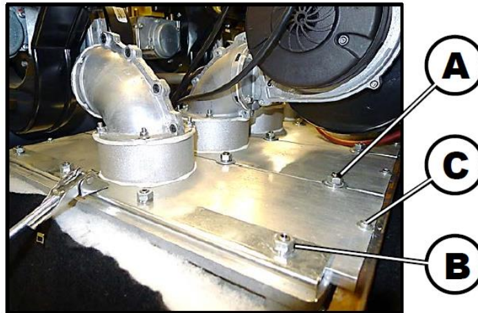
Figure 8-14: Removal of Burner Plate Hardware (Steps 9, 10, 11)
