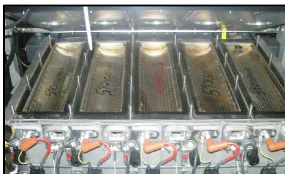
Figure 8-23: Burner Modules Exposed for Cleaning
