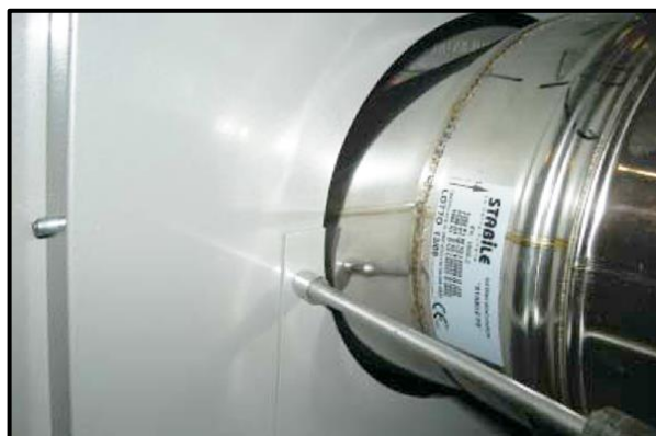
Figure 8-6: Remove Panels (Step 3) Figure 8-7: Remove Flue Assembly (Step 4)
