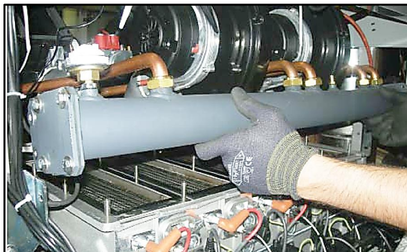
Figure 8-20: Lifting Burner Assembly from Front (Step 15)
