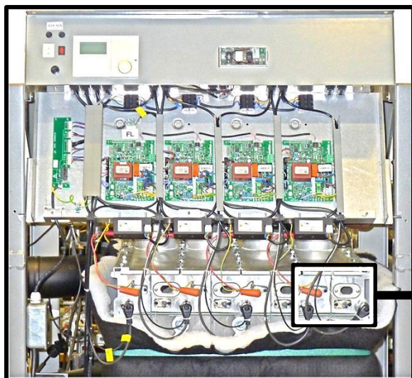
Figure 8-2: Boiler Flame Observation Port Location
