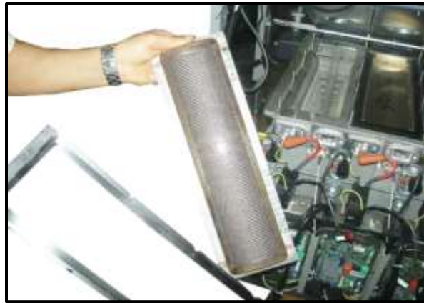
Figure 8-24: Removing Individual Burner Module and Gasket (Step 1)
