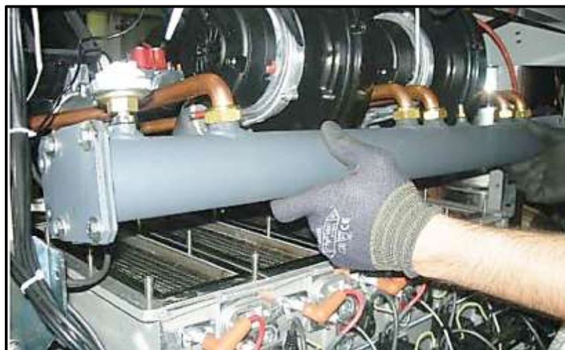
Figure 8-20: Lifting Burner Assembly from Front (Step 15)
