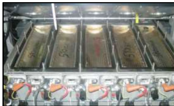
Figure 8-23: Burner Modules Exposed for Cleaning
