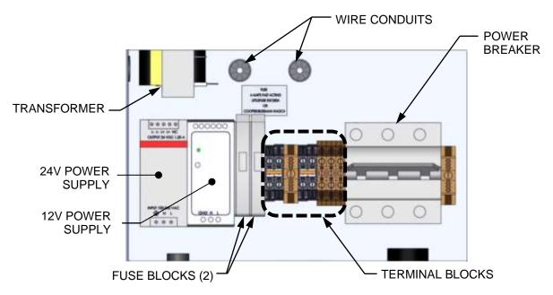
Figure 2-10c: BMK 2500/3000 Power Box Internal Components
