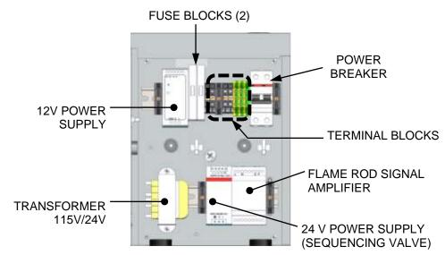
Figure 2-10a: BMK 750/1000 Power Box Internal Components
