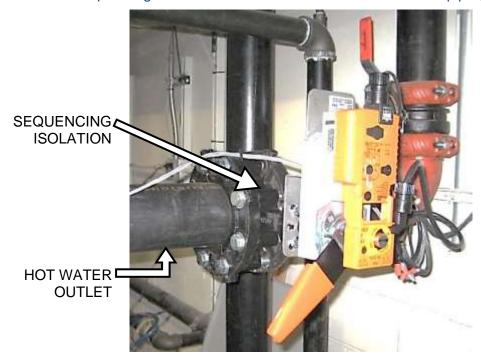
Figure 2-16: Sequencing Isolation Valve Installed
